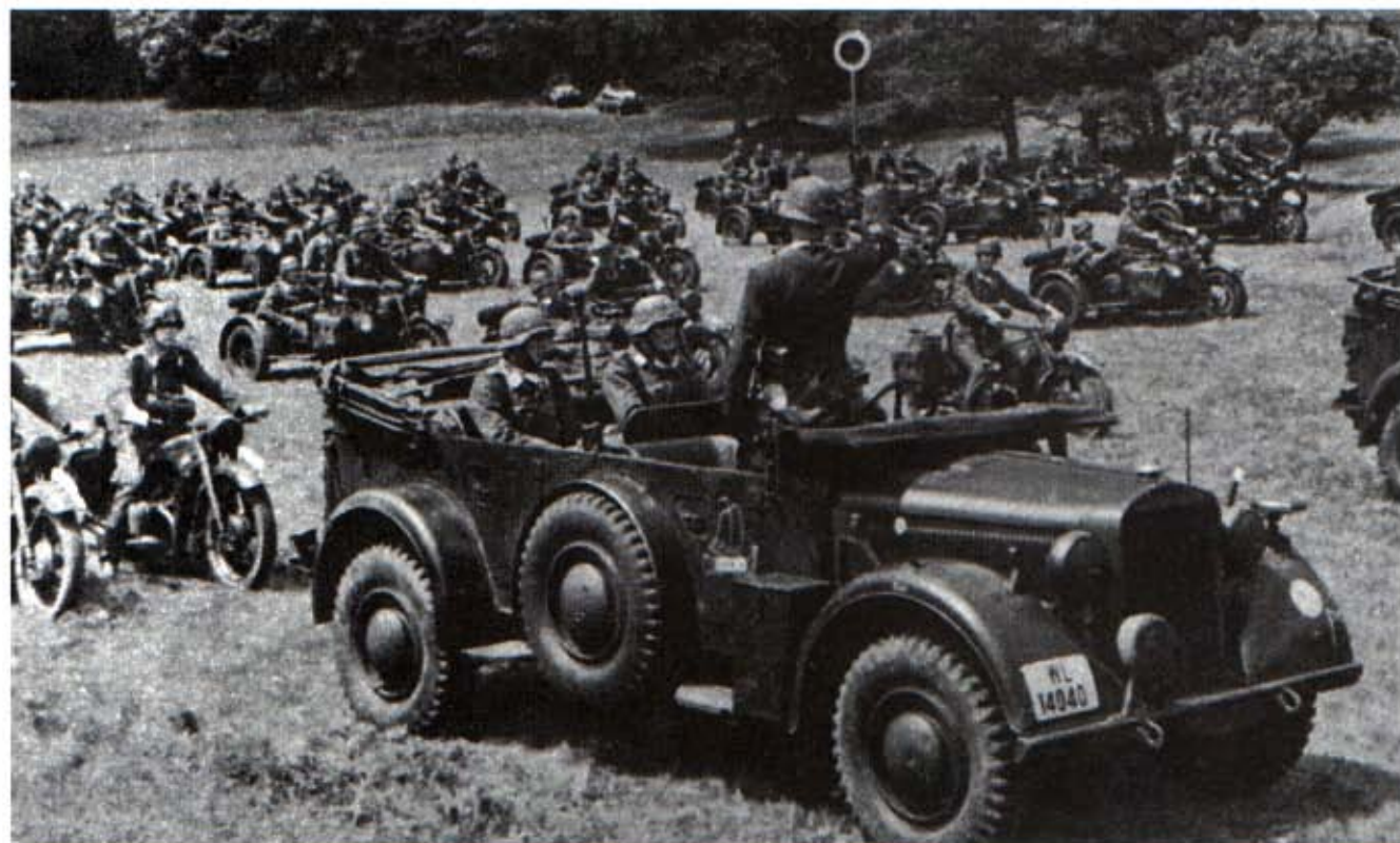
Below: The Mittlere Einheits Geländegängige Personenkraftwagen was made by two divisions of the Auto Union Group, Horch and Wanderer. Engines were 3.5 and 3.8-litre Horch V8s, or a 3.6-litre Opel six. (Bart Vanderveen Collection)
