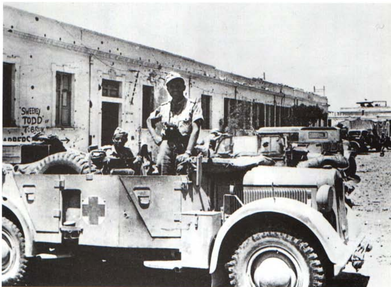
Above: This Horch m.gl. E. Pkw was among the first German vehicles to enter Tobruk in June 1942. Unusually, the spare wheel is carried inside the vehicle, not in an inset panel on the body side. (IWM)
