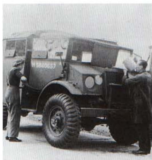
Above: Six-wheeled trucks of CMP pattern were made with either 6x4 or 6x6 wheel-drive. This is a Chevrolet C60X 6x6 van used by the Royal Canadian Electrical & Mechanical Engineers as a mobile testing station for equipment such as starters and generators. Behind the driver's door are two small doors covering the ventilator for the generator engine. (Public Archives of Canada)
