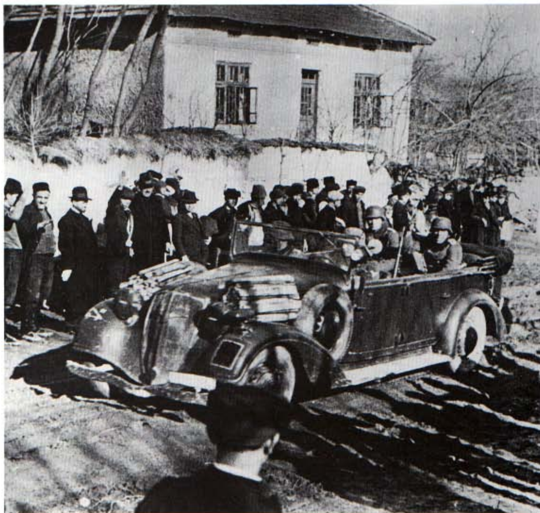
Below: An early 1930s Kübelwagen on the Mercedes-Benz 260 chassis, with body by Gaubschat. Later versions had doors. (Daimler-Benz)
