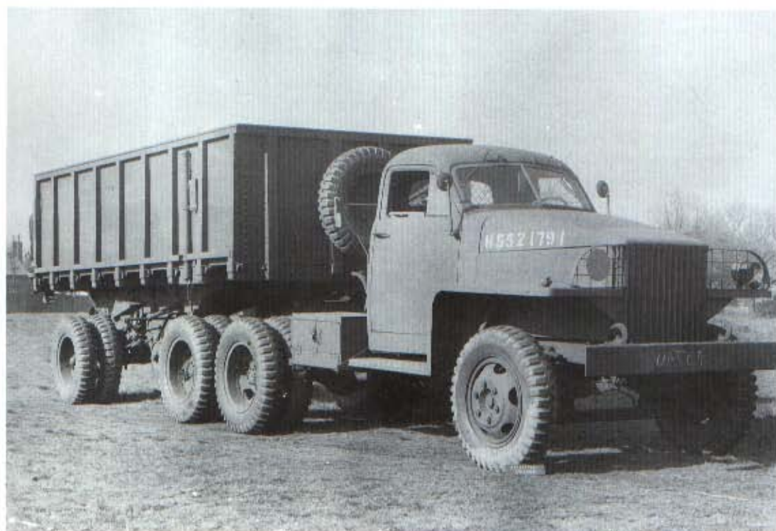
Left: Studebaker made nearly 200,000 trucks of similar pattern to the CCKW, though their engines (Hercules JXD) were larger at 5.2-litres. This is a relatively rare 6x4 tractor/trailer unit, rated for a 5 ton load, of which 8640 were made. A high proportion of wartime Studebaker trucks went to Russia. (IWM)
