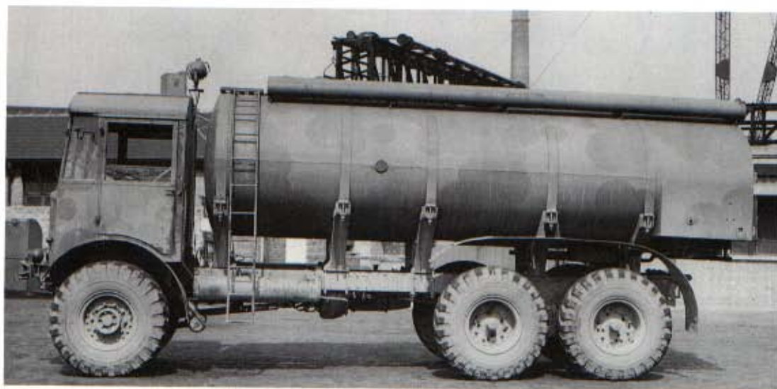
Left: The AEC 854 (0854 when fitted with diesel engine) was a 6x6 truck derived from the Matador 4x4 artillery tractor. Most were supplied to the RAF with 2500 gallon refuelling tank bodies, as here. Others carried mobile oxygen/nitrogen bodies, or Coles Mark VII petrol-electric cranes. (Nick Baldwin Collection)
