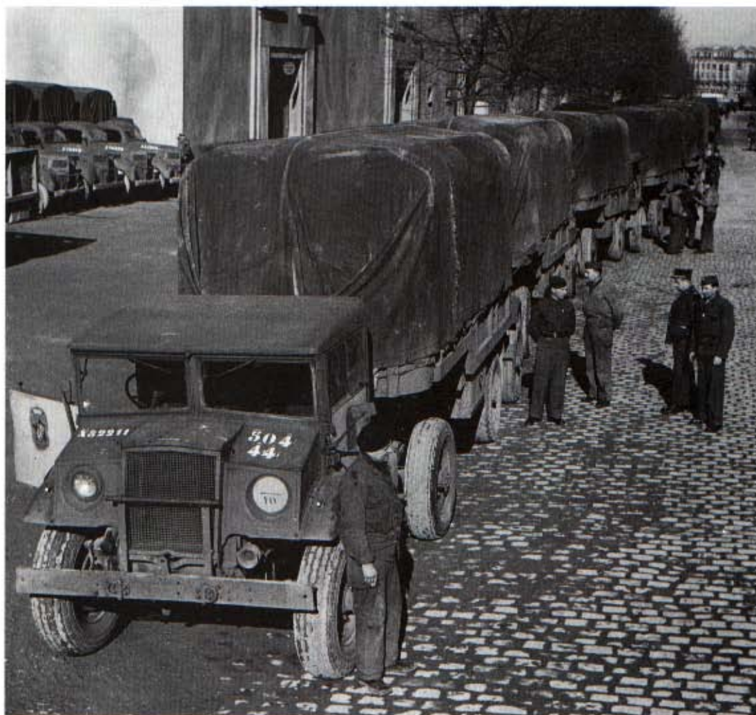
Left: Tractor/Trailer versions of the CMP range were known as F60T. The tractor was on a 115-inch wheelbase, and the trailers were non-detachable. They were rated for a 6 ton payload. Photographed in February 1945 this column is about to move out from the Porte de Versailles, Paris, to collect food supplies from a depot outside the city. The trucks were operated by French Army Transport Regiment. (IWM)
