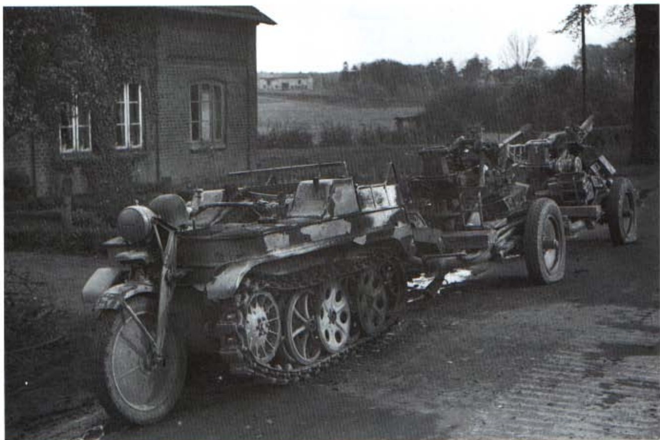
Above: NSU Kettenkrad towing two Flak guns, abandoned during the German retreat near Lubeck, May 1945. These machines were officially known as Kleines Kettenkrad (small tracked motorcycle). A total of 8345 were made between 1940 and 1944, by NSU and Stoewer. (IWM)
