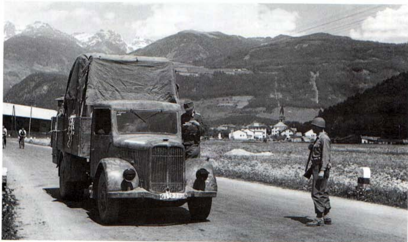
Above: One of many basically civilian designs which conformed to the Autocarro Unificato programme was the OM Taurus, produced under licence from the Swiss Saurer company. This photo, taken on 14 May 1945, shows a German soldier checking a German-operated Taurus during the round up of German troops in Italy on 14 May 1945. It was a most unusual situation; an American (right) and a German soldier patrolled together, the German stopping German vehicles and the American, Allied vehicles.
