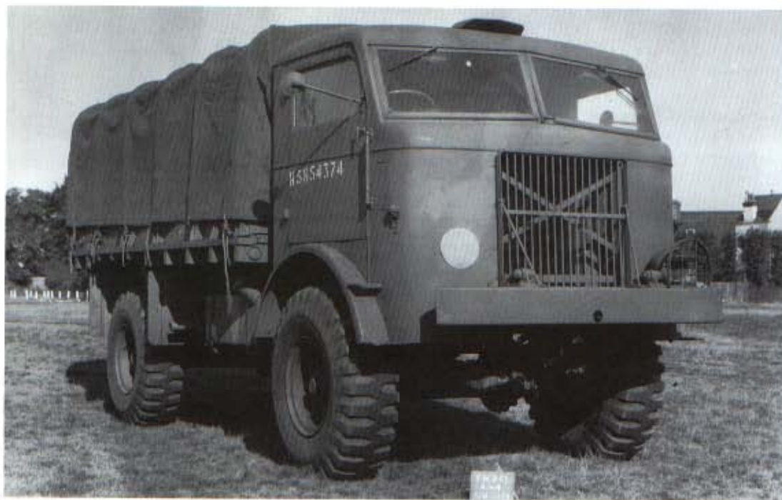
Left: More familiar to British troops than to American was the FWD SU-COE, a 4-ton 4x4 which was provided in large numbers under lend-lease. As well as the GS truck illustrated, the SU-COE was used as an artillery tractor and snowplough. (IWM)
